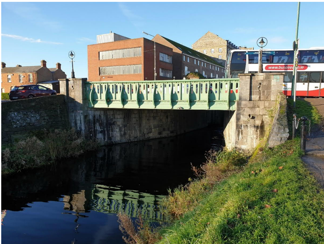
East elevation of existing Cross Guns Bridge – Location of proposed Ballymun 03
